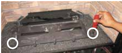
Diagram 1: Remove the left and right screws.
