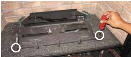
Diagram 1: Remove the left and right screws.
