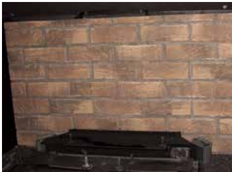
Back Panel Installed
