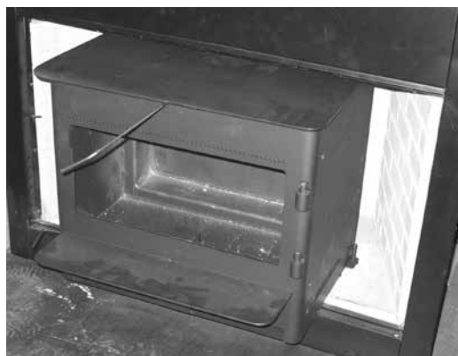
Diagram 5: Pull Rod In Place
