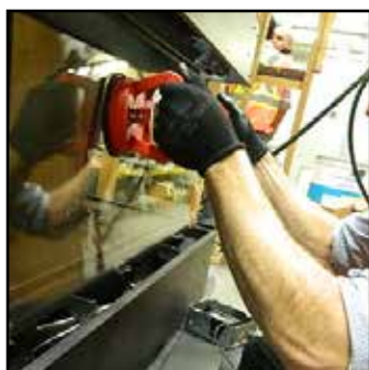
Handle glass with supplied vacuum clamps
