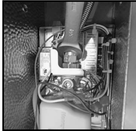
Figure 37: Removing gas connection.
