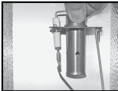
Figure 17: Spark igniter with its ignition wire and ground wire.
