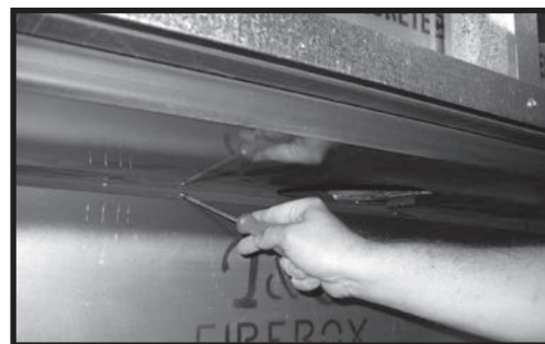
Figure 38: Securing top porcelain panel.
