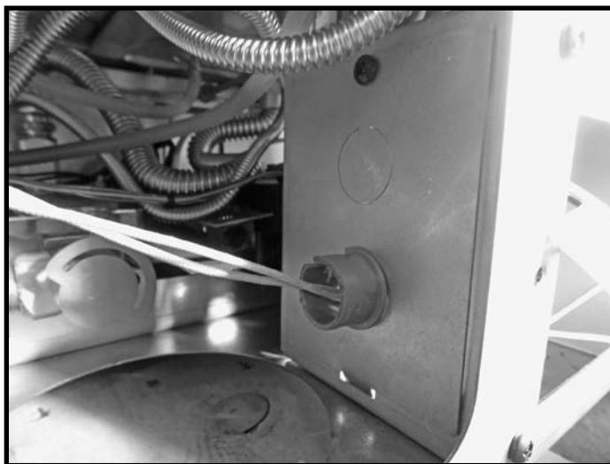
Figure 80: Threading wires through knockout.
