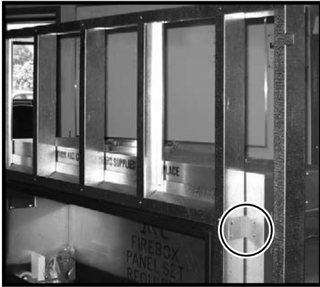
Figure 20: Bend tab out 90 degrees.
