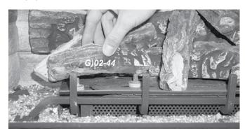
**10)** Place the embers and Rockwool on the exposed front burner tray.
